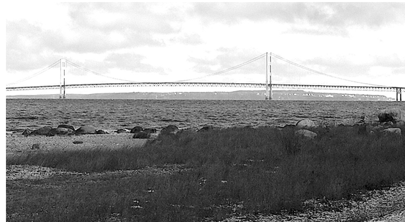
In accordance with Gov. Gretchen Whitmer and Michigan Department of Health and Human Services' recommendations designed to help prevent the spread of Coronavirus Disease 2019 (COVID-19), the Mackinac Bridge Authority (MBA) will not accept cash transactions. Photo by Jim Akans
